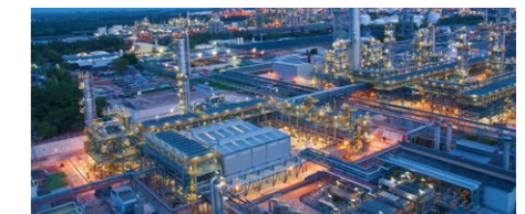
Industrial Park Process Water
