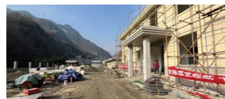
Water Plant Expansion & Upgrades
